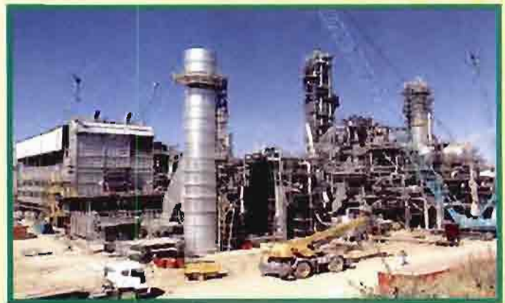
A view of Algeria Oman Fertilizers project site at Arjew, Algeria
