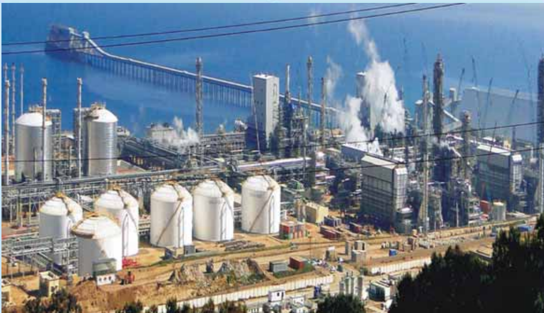
Construction Site of Algeria Oman Fertilizers Project, Algeria
