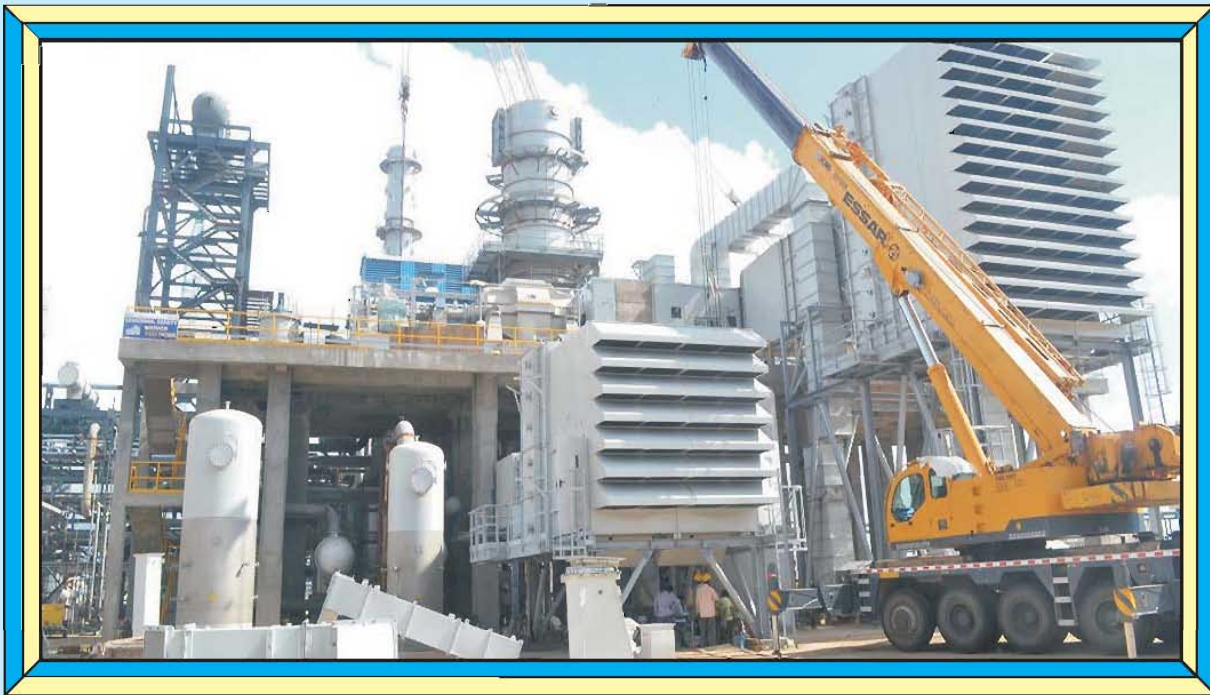
A View of Matix Fertilizers and Chemical Project, Panagarh, West Bengal.
