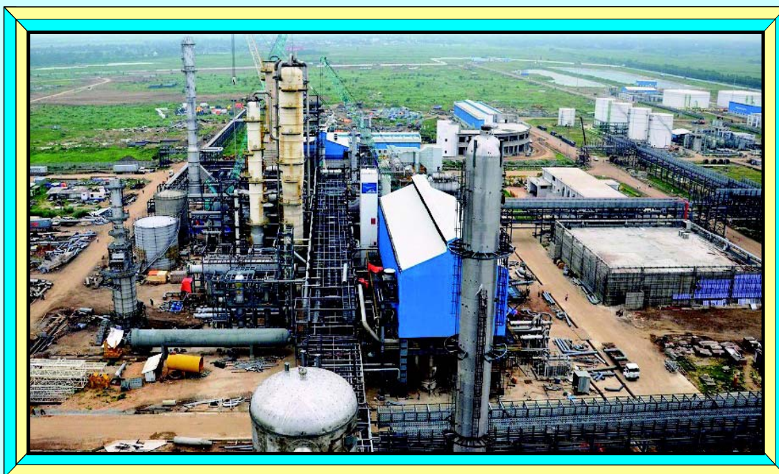
A View of Matix Fertilizers and Chemicals Project Site
