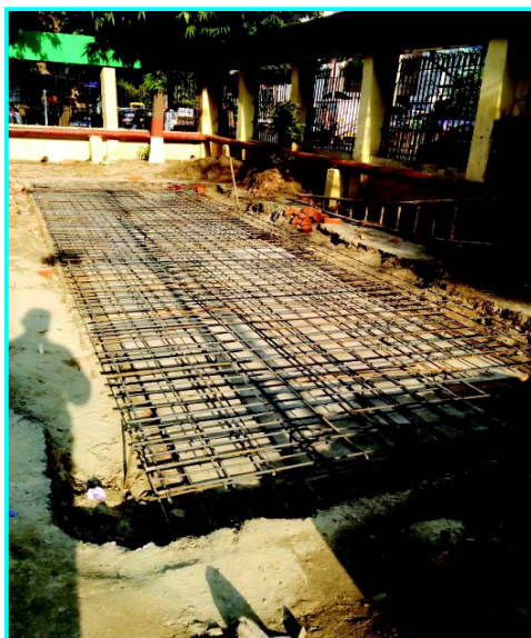
Rain Water Harvesting System at PDIL Noida
