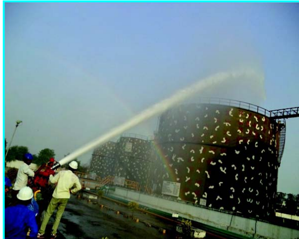
PMC services for HPCL Terminal Automation
