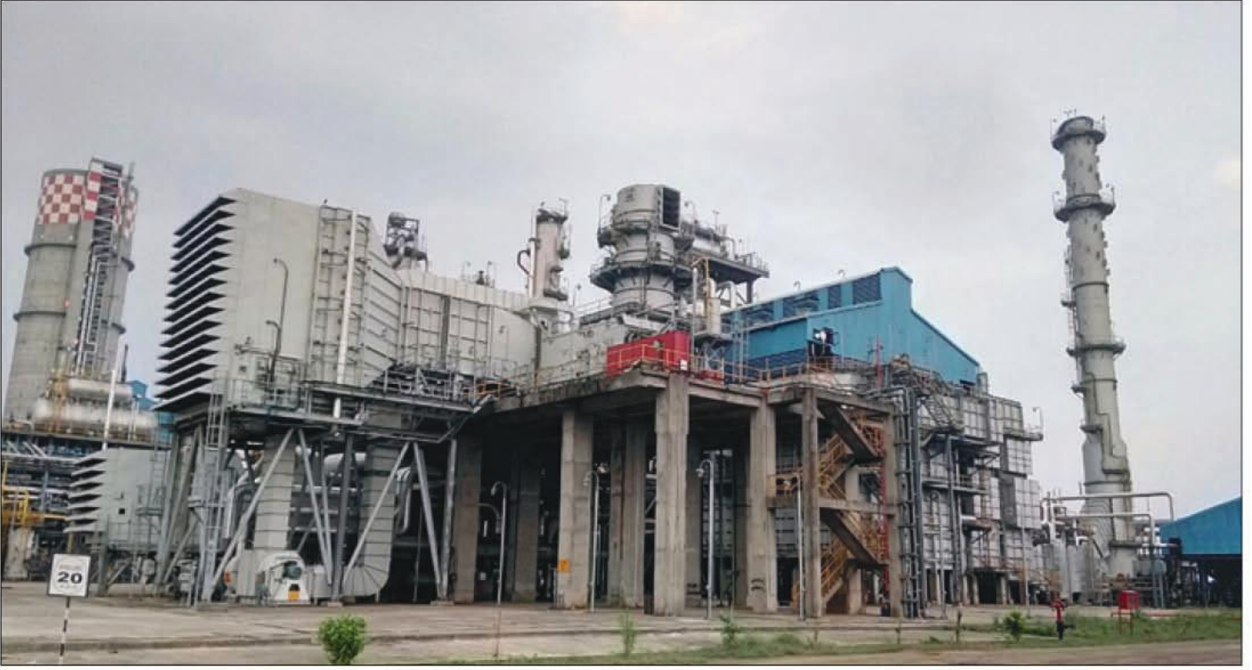
A view of Matix Fertilizers plant executed by PDIL.
