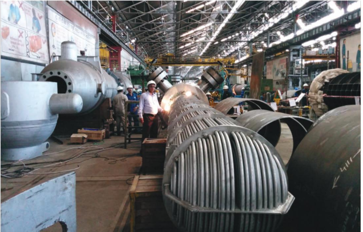
Leakage checking between tube sheet and tube bundle of ammonia pre heater for RCF Thal
