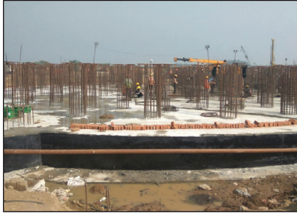
Ammonia Storage Tank-B under Construction at HURL Gorakhpur
