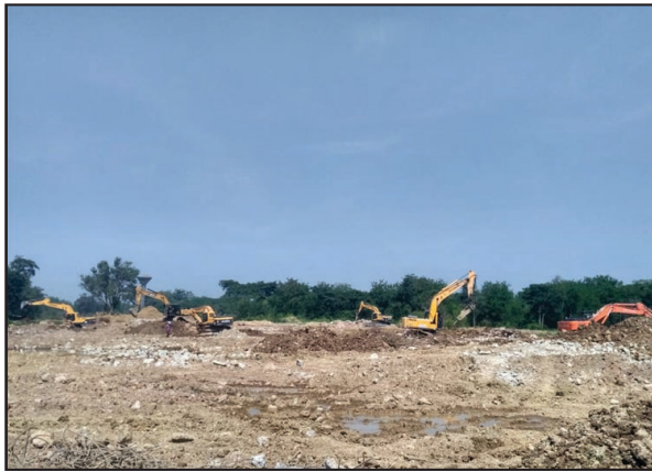
Site Activities at Talcher Project
