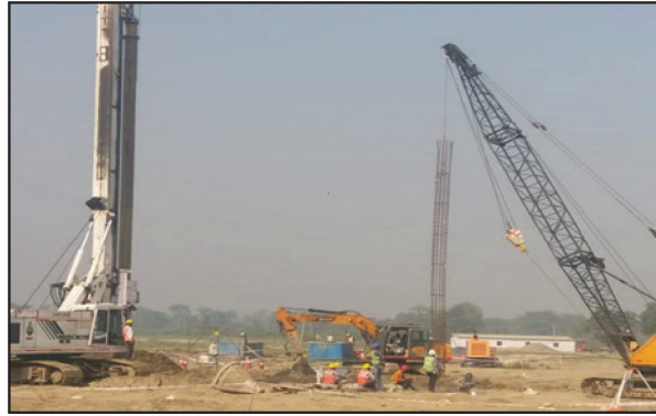
Piling Work in Ammonia Pipe Rack Area of HURL Barauni
