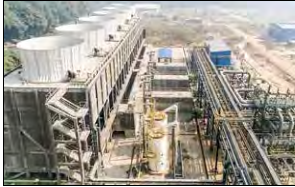
HURL-Gorakhpur- Urea Cooling Tower
